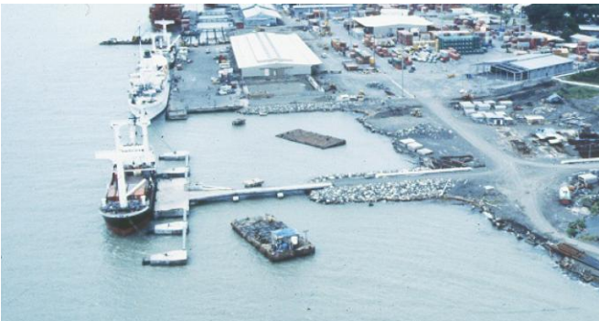
LAE PORT TANKER BERTH, Papua New Guinea (AECOM)
